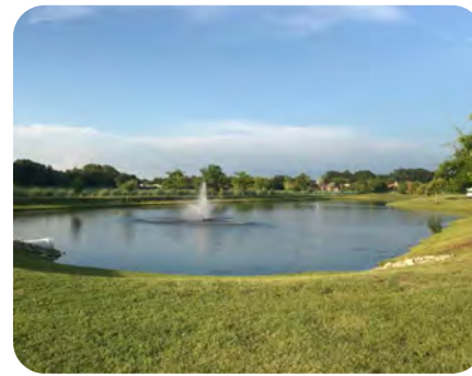
Runoff Capture and Reuse
