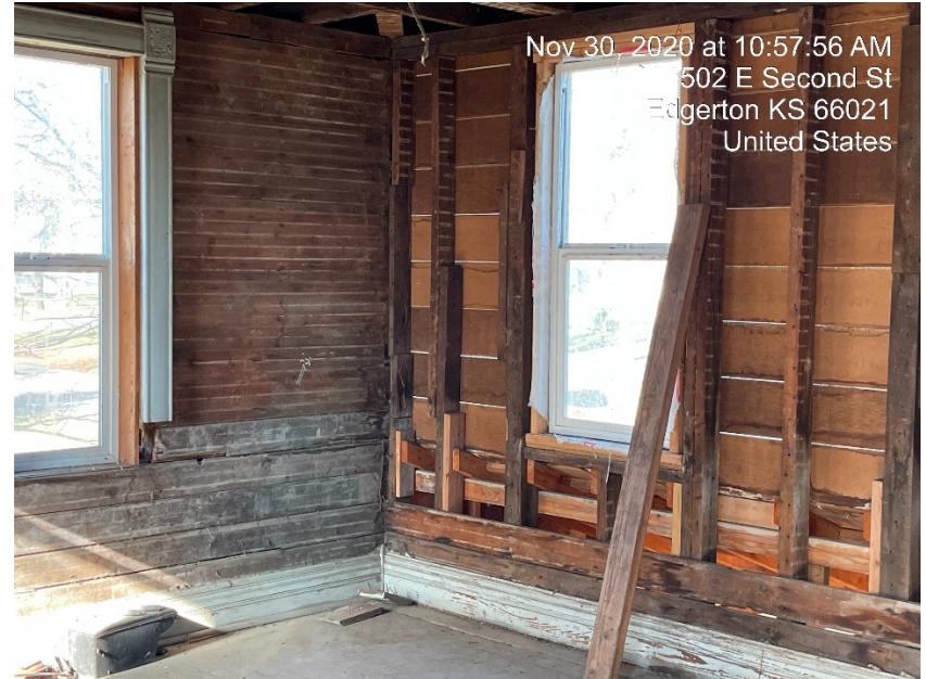
Upstairs bedroom - exterior sheathing and siding to be replaced.
