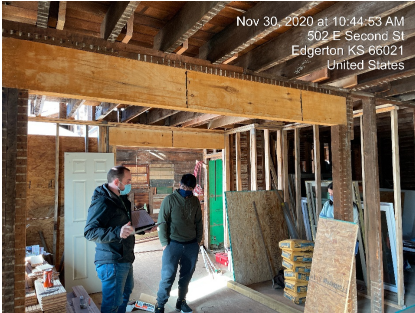
New header beams to support second floor – interior doorways.
