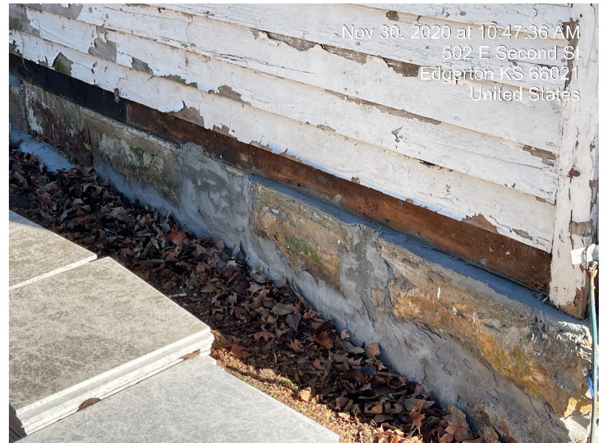
Additional foundation tuck pointing.
