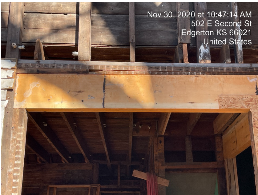
New header beam to support second floor – exterior doorway to deck area.
