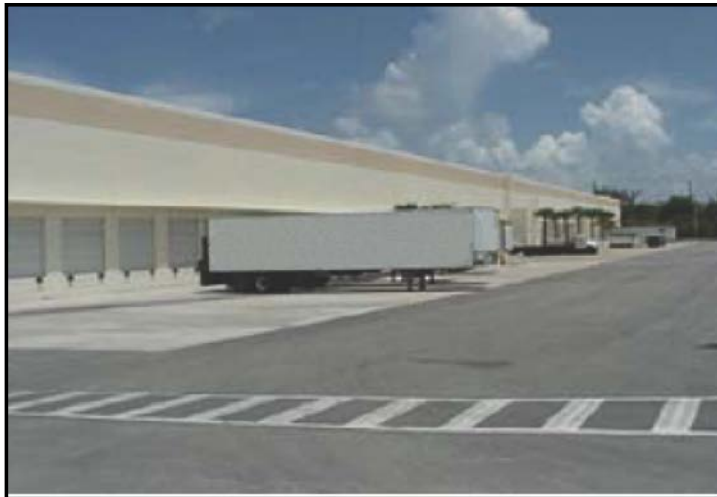
Figure 2. Typical Loading Dock
