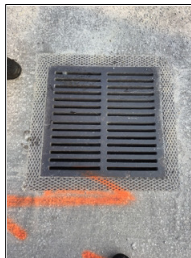
Figure 16. Structure Condition: Could Not Inspect.
