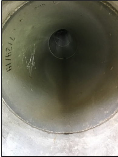
Figure 17. Pipe Condition: Excellent. New pipe. No visible defects, cracks, etc.
