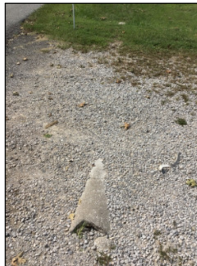
Figure 21. Pipe Condition: Failed. Invert of pipe has corroded away
