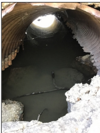
Figure 21. Pipe Condition: Failed. Invert of pipe has corroded away
