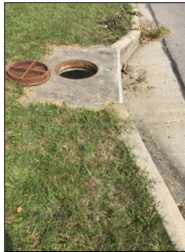
Figure 12. Structure Condition: Good.
