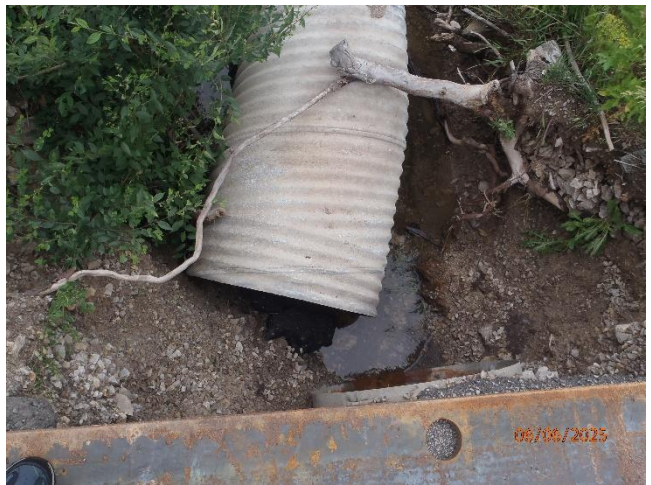
Fig. 4 – Drainage pipe has separated
