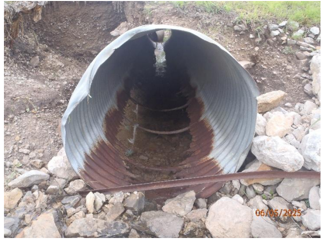
Fig. 2 – Bottom of pipe has deteriorated away
