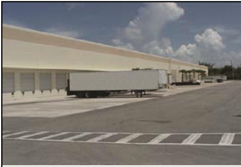
Figure 2. Typical Loading Dock
