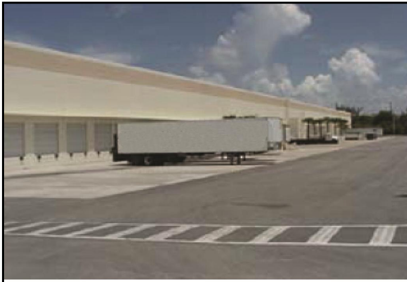
Figure 2. Typical Loading Dock
