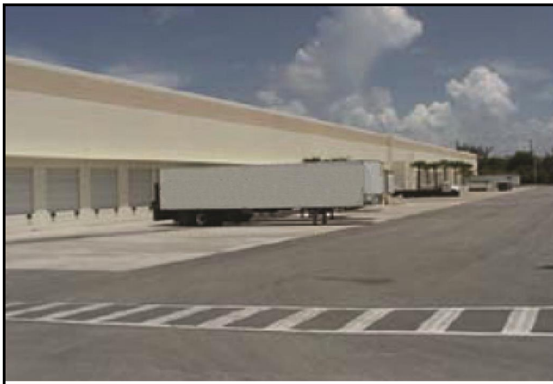
Figure 2. Typical Loading Dock
