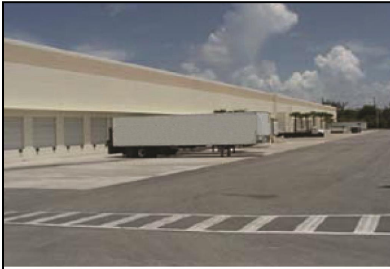
Figure 2. Typical Loading Dock
