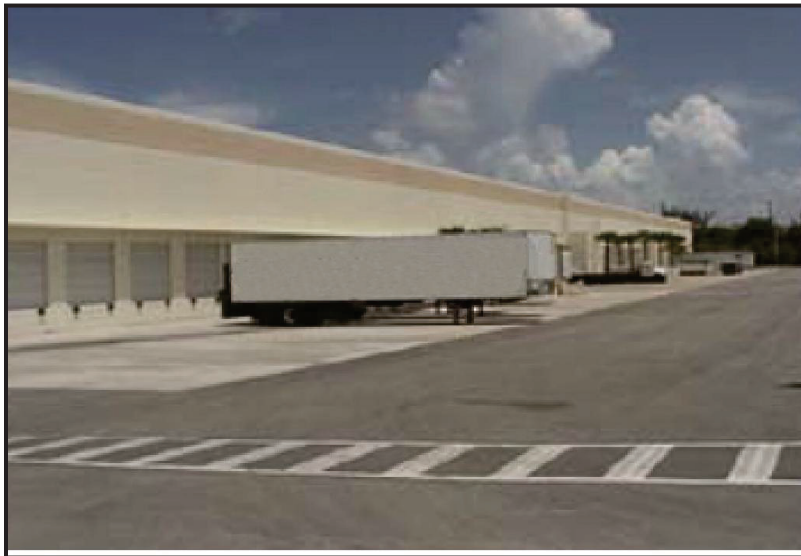
Figure 2. Typical Loading Dock
