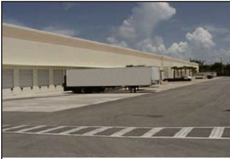
Figure 2. Typical Loading Dock
