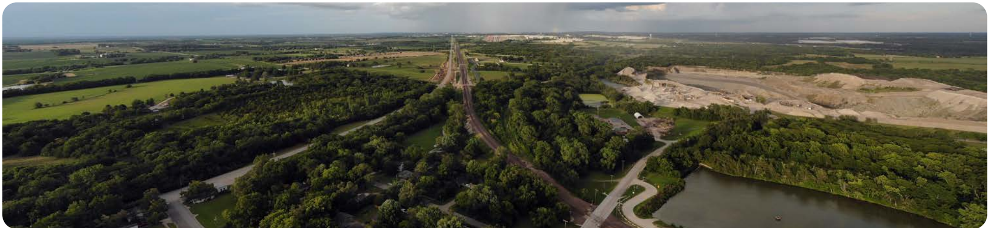
Aerial View of Edgerton, looking northeast towards the BNSF Intermodal Facility
