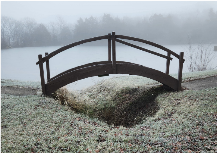
The bridge at Edgerton City Lake on a foggy and frosty winter morning.
