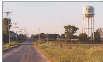
Edgerton Water Storage Tank
