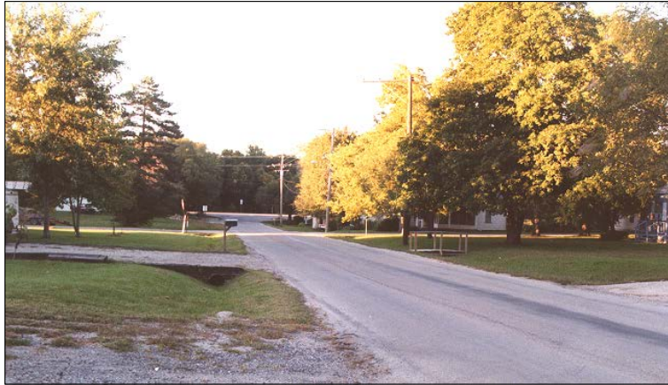
Open Drainage Ditch in Original Town Edgerton
