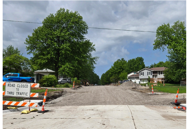
Gravel covers Edgewood before new asphalt is laid.
