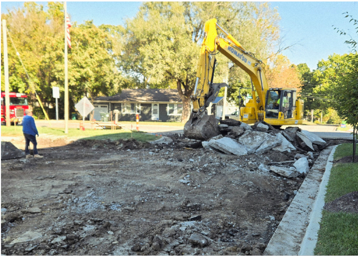
Road crews are working hard to make progress before winter arrives!
