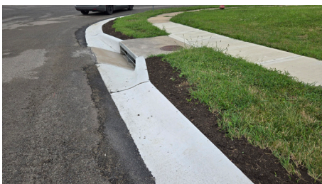
Concrete curb & gutter repairs
