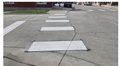
New pavement markings
