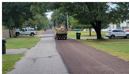
Chip-seal road treatment
