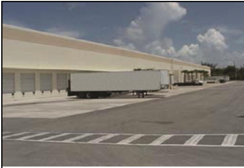
Figure 2. Typical Loading Dock
