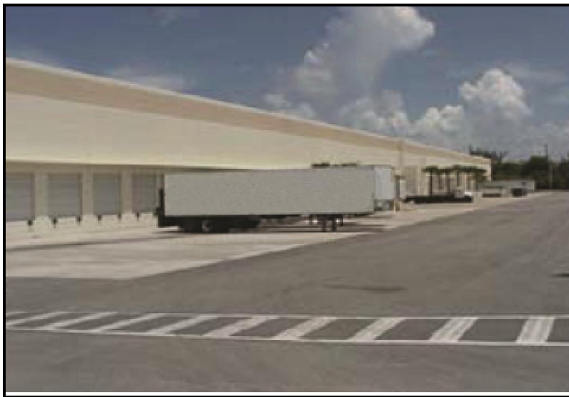
Figure 2. Typical Loading Dock
